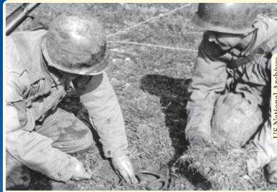
US engineers lay an anti-tank mine M1A1.
