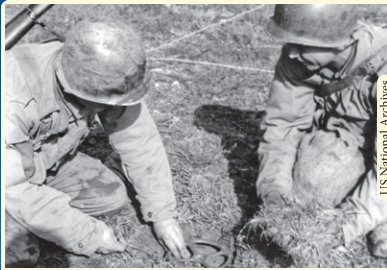
US engineers lay an anti-tank mine M1A1.
