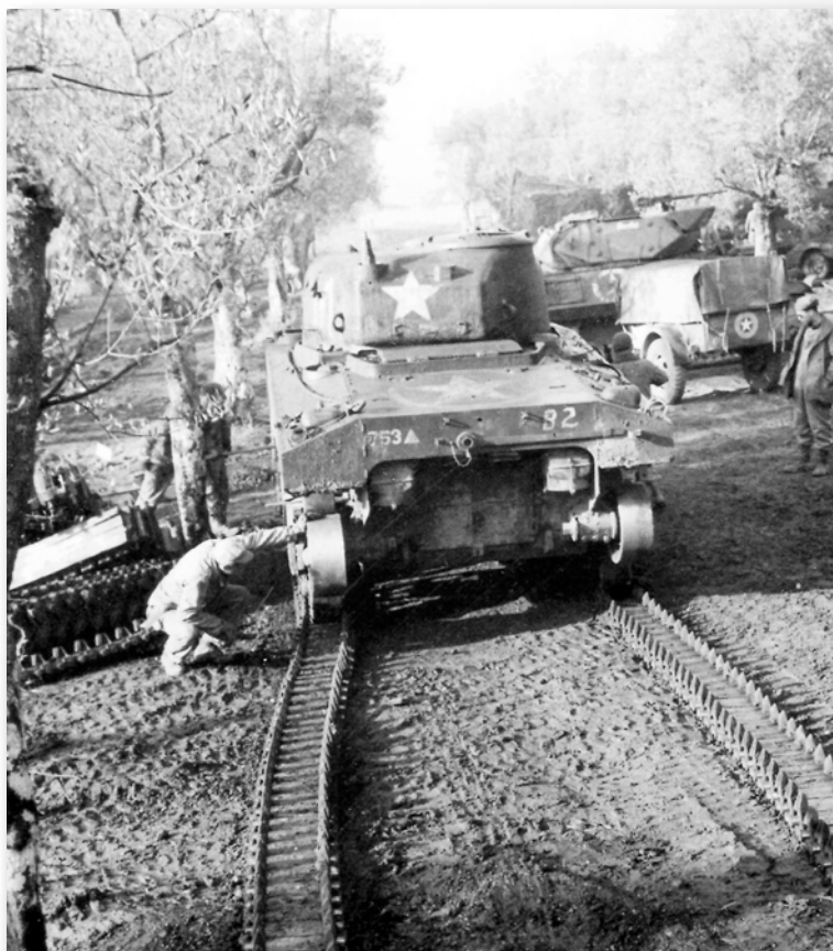
REPAIR OF TANK TRACKS IN THE FIELD US NATIONAL ARCHIVES
