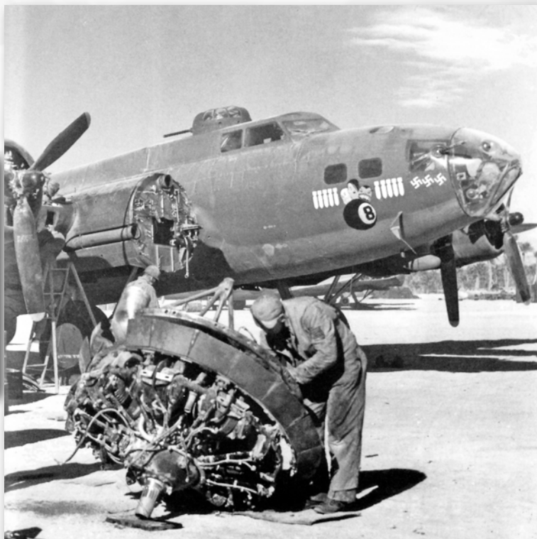
REPAIR OF A B-17 FLYING FORTRESS ENGINE US NATIONAL ARCHIVES
