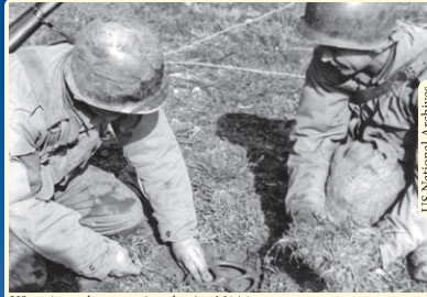
US engineers lay an anti-tank mine M1A1.
