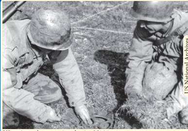
US engineers lay an anti-tank mine M1A1.
