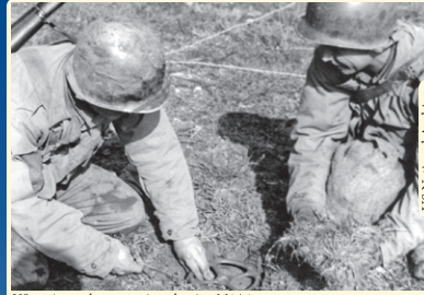
US engineers lay an anti-tank mine M1A1.
