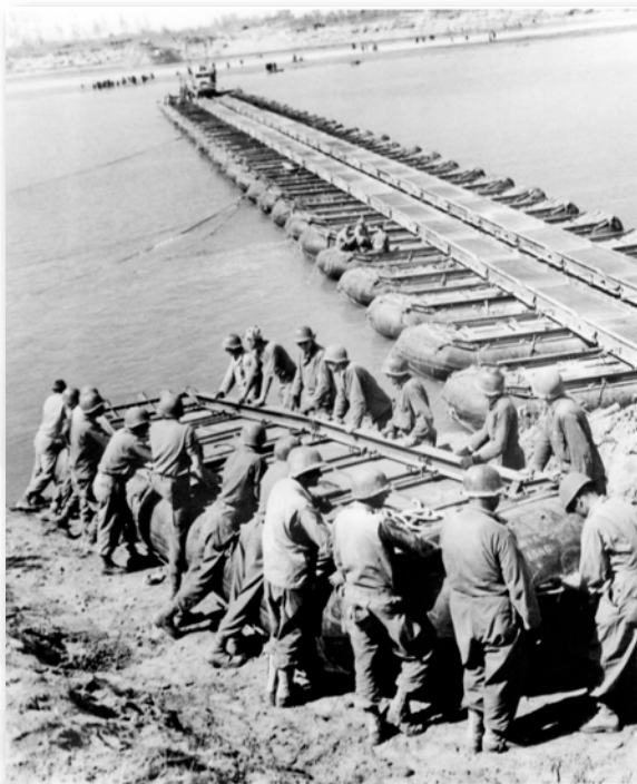
US COMBAT ENGINEERS CONSTRUCT A PONTOON BRIDGE US NATIONAL ARCHIVES
